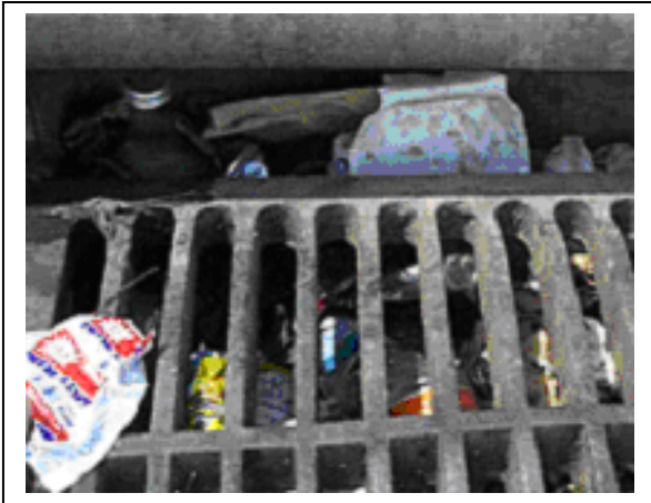
Litter filling the sewer grates in Pittsburgh.
