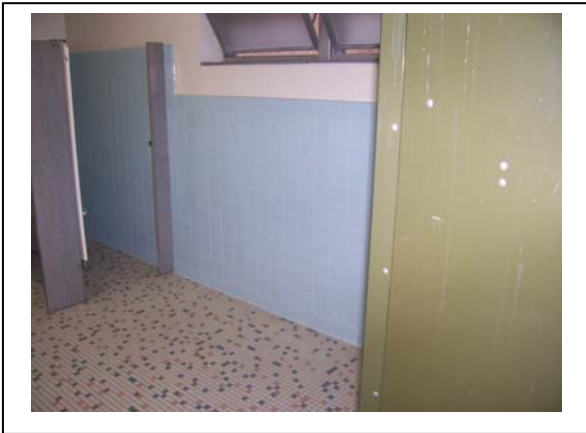
Photo 1: Women's restroom, pre-installation.
