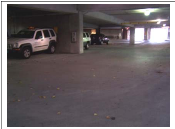
ASU Parking Deck with unmarked L-turn
