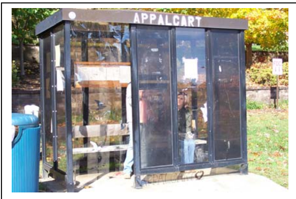
Vinyl curtain protecting students from weather conditions.
